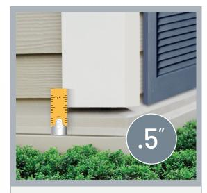
• At least ½" above brick, concrete or flashing to allow for water drainage.
